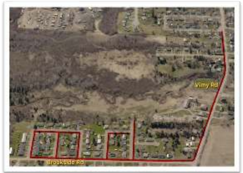
Sidewalk renewal on Brookside Road and Vimy Road
