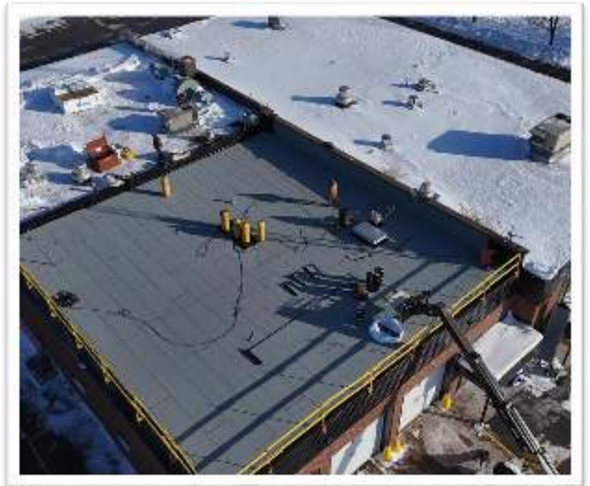
Partial roof replacement – 69 Pictou Road
